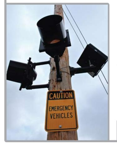
The system also allows for portable activation of the beacons from inside a vehicle, thanks to an optional secondary master controller, and programmability features allow users to determine how long the beacons should flash before automatic shut-off.
